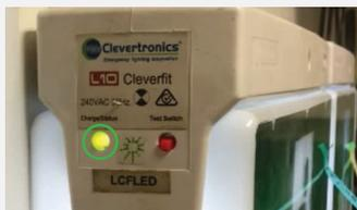
This sequence shows that the fitting passed its last test and has reverted to the normal standby state. At this point, you can simply walk the site and look for fittings flashing the Amber or Red failed indications as shown on the next page and know that all other fittings have passed.
